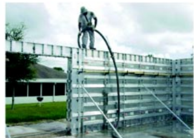
High strength design mix concrete used in walls.
