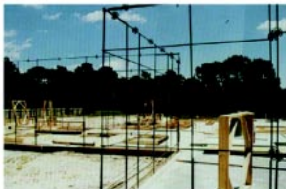
Reinforcing steel is anchored to the foundation.
