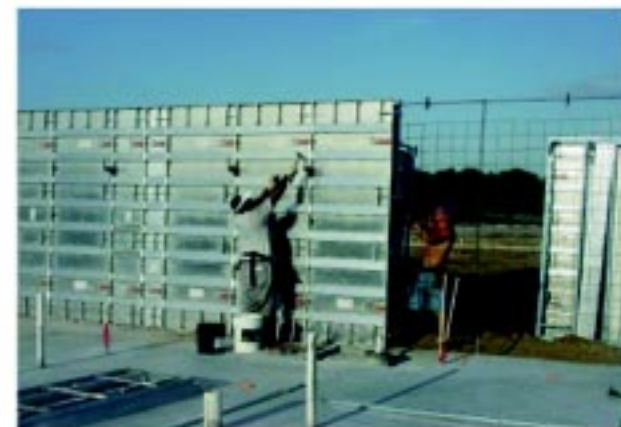
Aluminum forms insure high quality construction.
