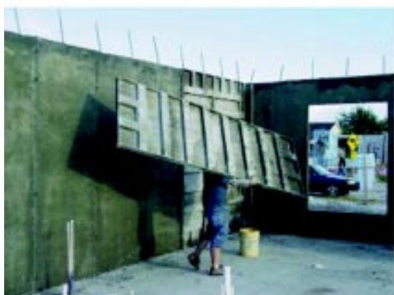
Reinforcing steel is anchored to the foundation.
