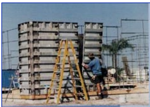
A metal form panel is installed for a CIP concrete wall.
