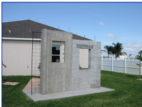
A mock-up of the Mercedes Homes cast-in-place concrete wall next to a standard cmu wall.
