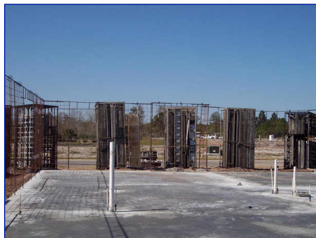
Mercedes Homes raises the reinforcing steel for their next cast-in-place concrete wall home. (Source: Mercedes Homes)
